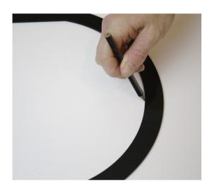
Draw a line inside the collar to mark the hole cut needed. If you wish to cut a perfectly circular hole, move the fitting ring round to ensure a circle is drawn all the way round.
